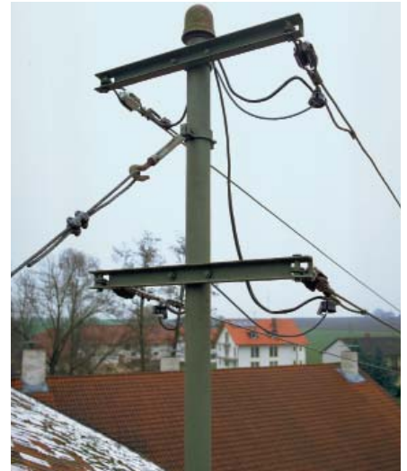
Service entry through overhead system
