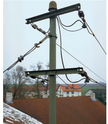
Service entry through overhead system
