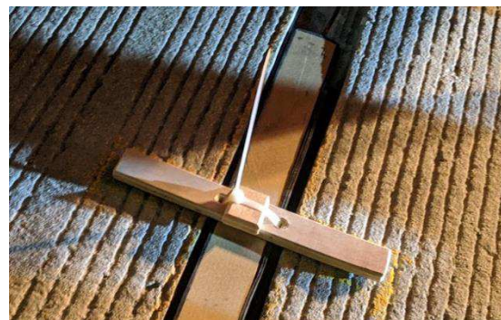
Figure 6. Attachment and Use of Mounting Brackets
