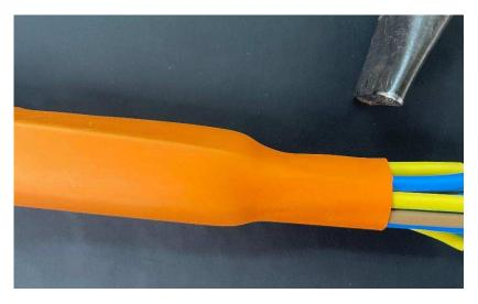
c. Work progressively to the end of the tubing ensuring uniform heat application. This can be achieved by either rotating the assembly or the heat gun. See figure 2. Ensure there is no air entrapment inside.
