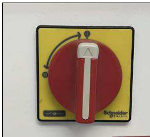
Figure 15: Main switch
