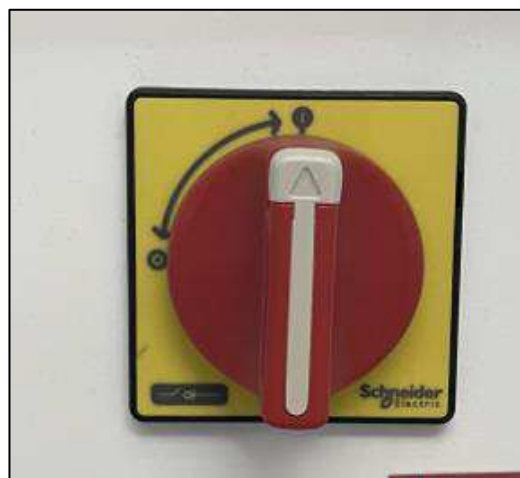
Figure 18: Main switch (example)
