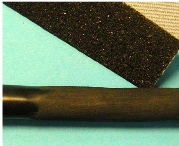
Figure 1 Degreasing cable jacket
