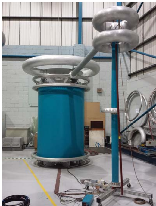
500 kV power transformer with PD and watt loss measurements
