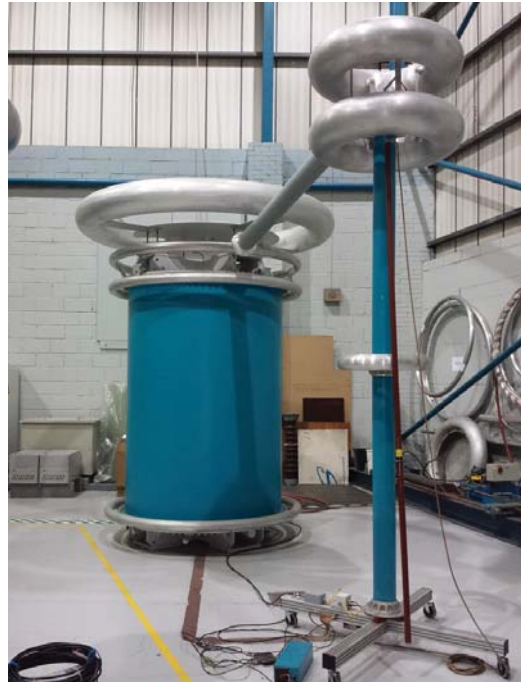
500 kV power transformer with PD and watt loss measurements
