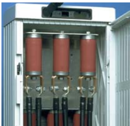
Cable sheath arresters
