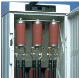
Cable sheath arresters
