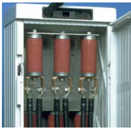
Cable sheath arresters
