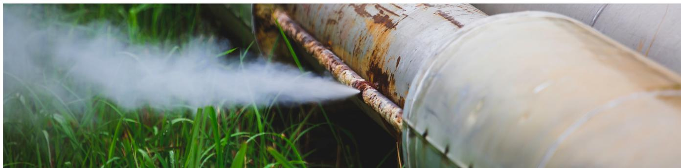
Fig. 1: Corrosive environmental conditions affecting an insulated pipe.
