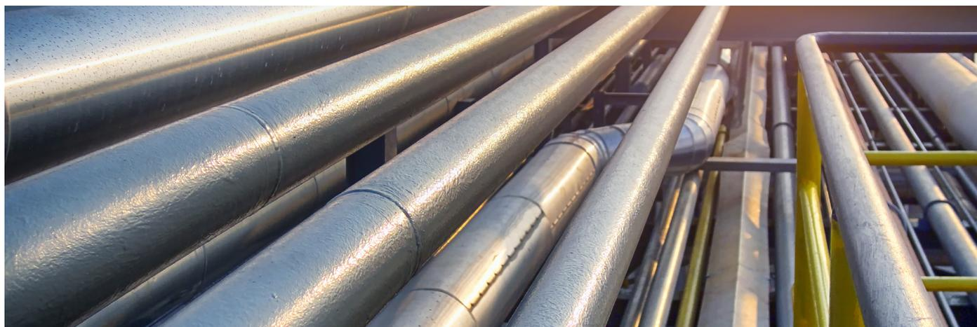
*Fig 2: Insulated pipe with metallic cladding.*
